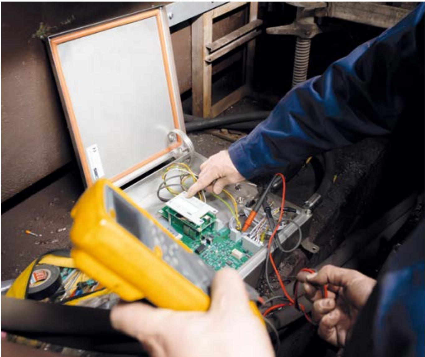
Figure 3: Installation of the EdgerKraft Controller (MMV) in a hot rolling mill
